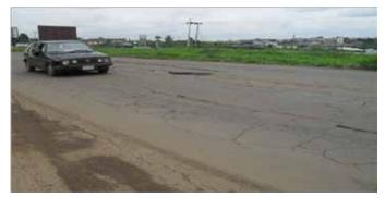
Plate 1: Typical Pavement failure along Lagos – Ibadan Expressway
